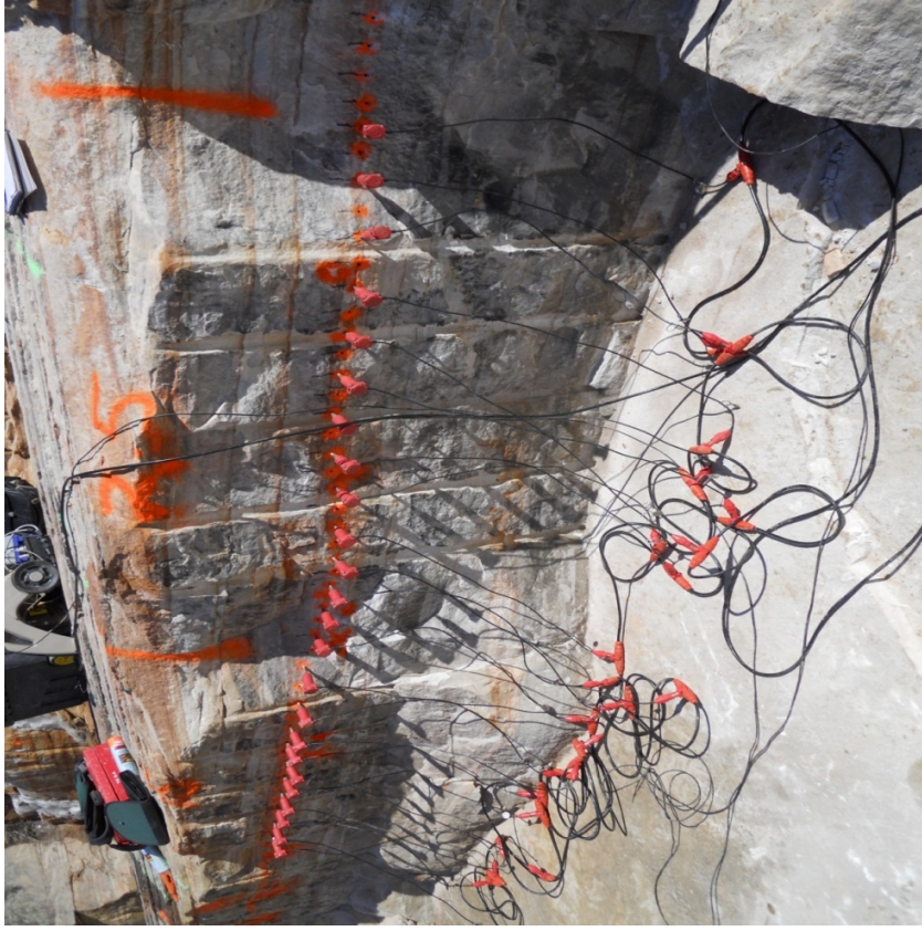
Figure 5.15: Shot areas 15 and 25 were adjacent blast sections together spanning over a 3.05 meters (10') wide area. They were both analyzed together using a 3.66 meters (12') array.
