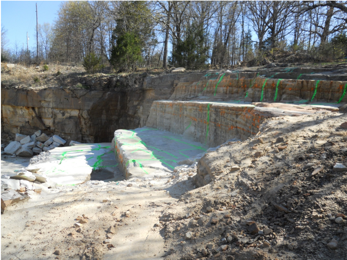
Figure 5.4: Safe workable benches were easily created without performing “lift” shots.
